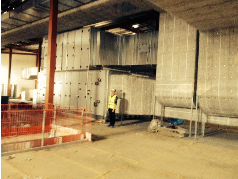
Figure 12: In the plant room above the cinema ten fan units, 10 tons each, is located, possibly causing structure borne noise and vibration.
